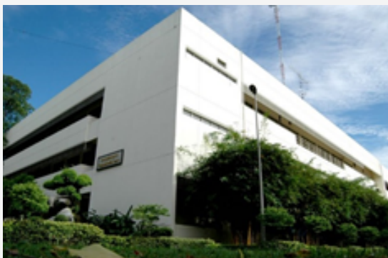
Less Glass Windows to Reduce Solar Radiation
